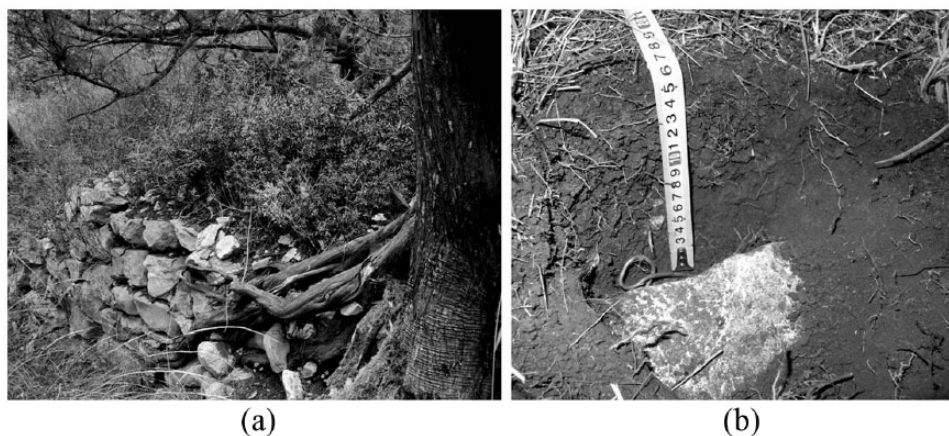
Figure 2. The Roman fortress of Charax (AD 1st–mid-3rd centuries): (a) fragment of the lower defensive wall (left) and (b) soil section (no. 10) atop the defensive wall (right).
