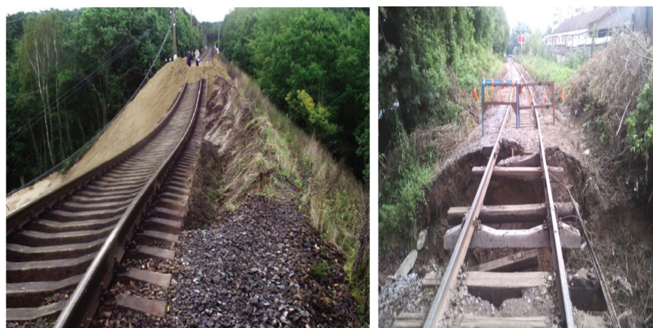
Figure 1. Sudden destruction of the railway roadbed as a result of natural factors.
